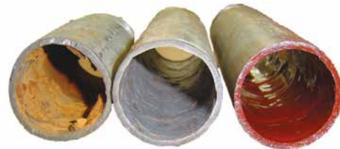
Pipe before cleaning, after cleaning, and after lining with Nu Line.
